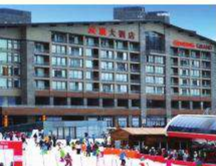
Genting Hotel, Zhangjiangkou, Hebei, China
