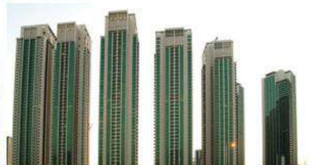
Reem Island Residential Apartment, Abu Dhabi
