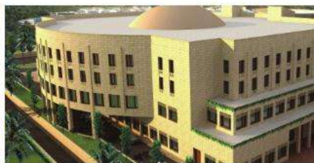
New Sindh Assembly Building, Karachi, Pakistan
