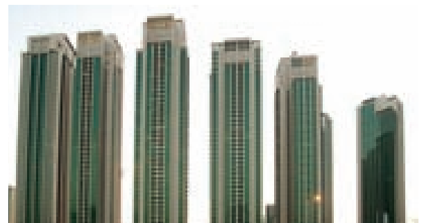
Reem Island Residential Apartment, Abu Dhabi
